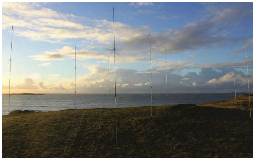
Rich, GM3PPG's 9 element 80m phased vertical array on the west coast of North Uist.
